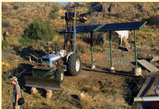
Figure 20: Solar panels for the electric pump at the new well. Picture: J. Heinzmann.
