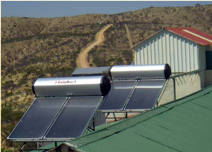
Figure 4: The sun's radiation heats up the water in the solar heaters. Picture: J. Heinzmann.
